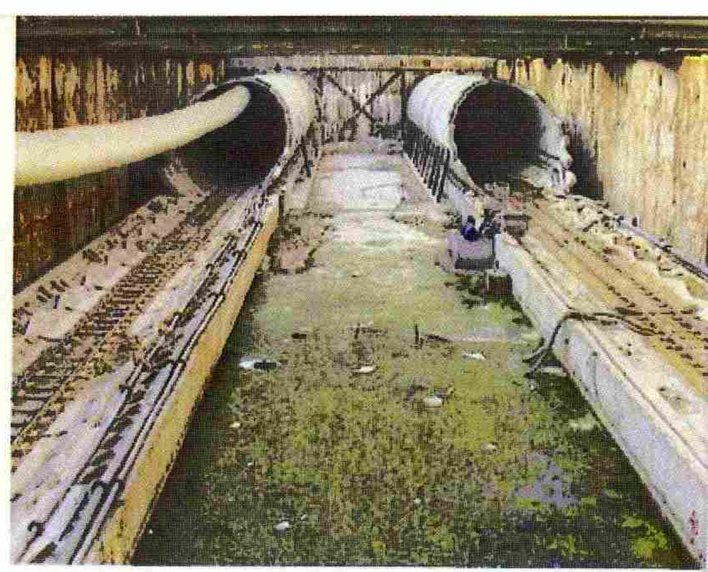
Concrete TBM cradles
