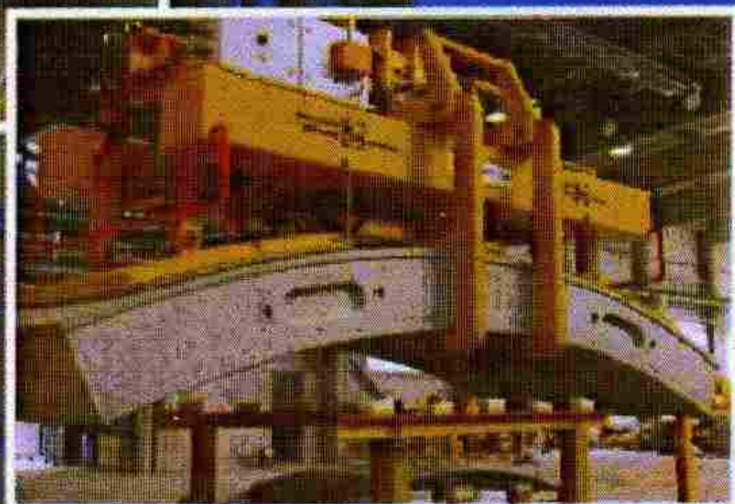
Segment handling equipment, Project Brenntunnel HB, Jenbach, Austria
